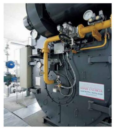
**STEAM MATIC SM are low consumption boilers:** Bono technology ensures a thermal efficiency of 89% reducing fuel consumption to the minimum. Additional devices such as flue gas/air, flue gas/water economisers or Integrated control system Optispark allow to reach 95%!
